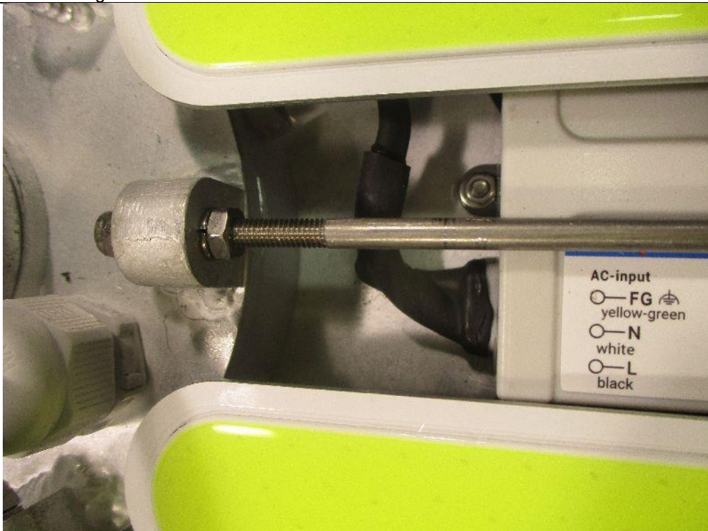
Bild / Picture 8: Securing of LED converter
